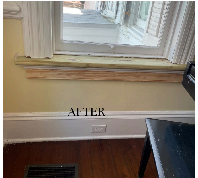
REPLACEMENT OF ROTTEN WINDOW WOOD
